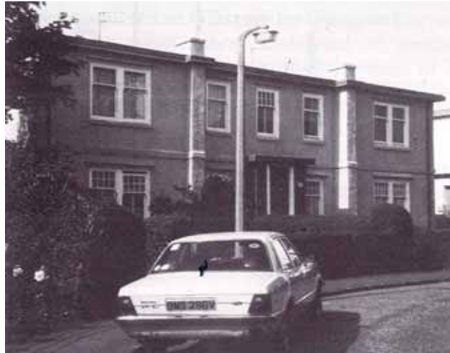
Figure 1.5 - A no-fines concrete house (Corolite)
