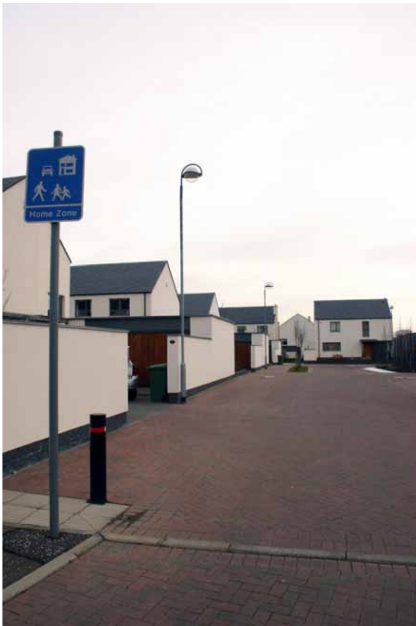
Figure 2.8 – The different approach to the plot edges creates multiple levels of interaction with the street.
